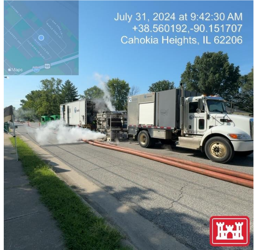
Curing Liner with Steam
