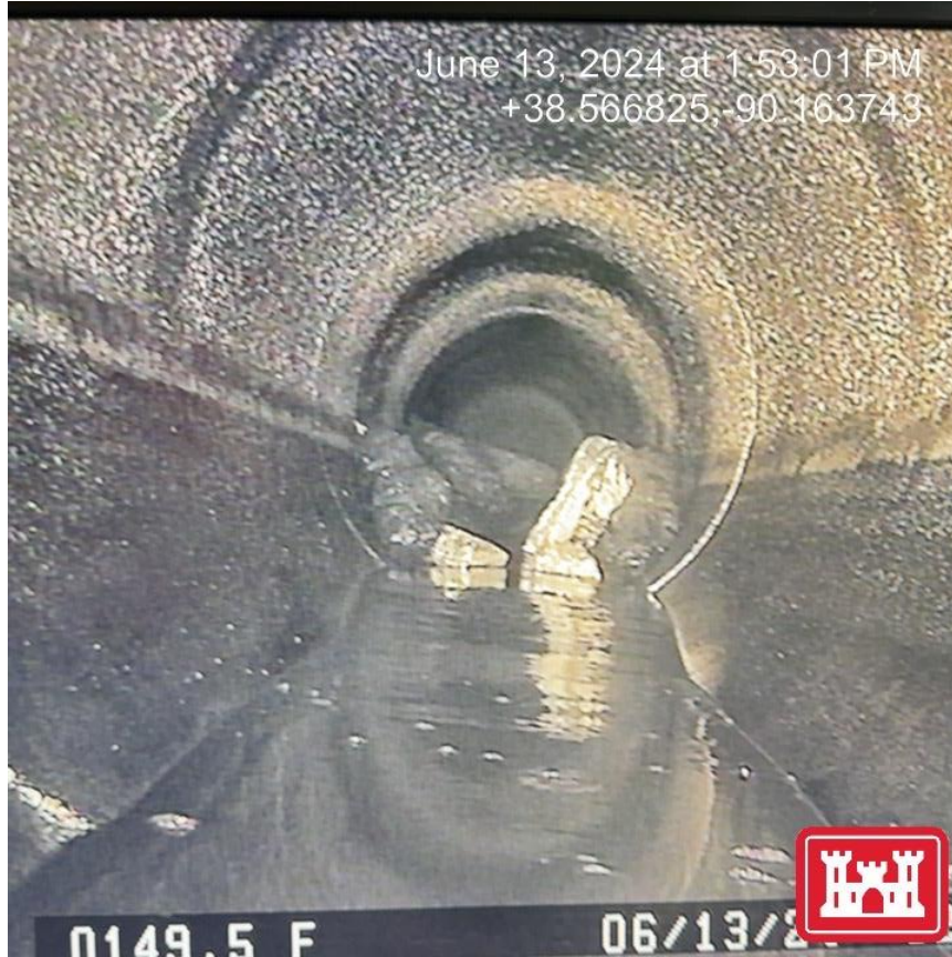
Live inspection & Cleaning
